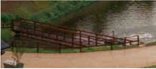
Inlet zone with scum baffle and walkway made of wood
